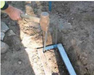
Next while holding the post vertical secure the 'diagonal' support brace into position (approx 2m from the ground) and then drive the stake into the ground in the appropriate position and adjust to level.
