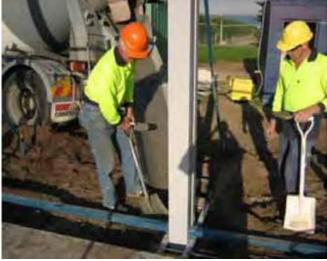
After the posts have set and the support shoes have been removed you should mix up a mortar mix and with a trowel slope the concrete away from the post for correct drainage.
