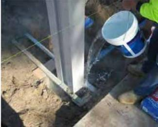
Go back and have one final check of all post alignments before pouring concrete and also check the alignment as you go.
