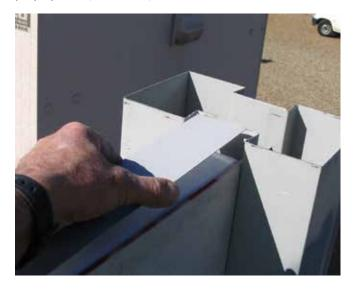
Next fit the wall capping (outlined further in the next step) + bracket and Tek screw in place. Make sure to 'pull or push' the post if required to achieve the correct alignment before Tek screwing off.
